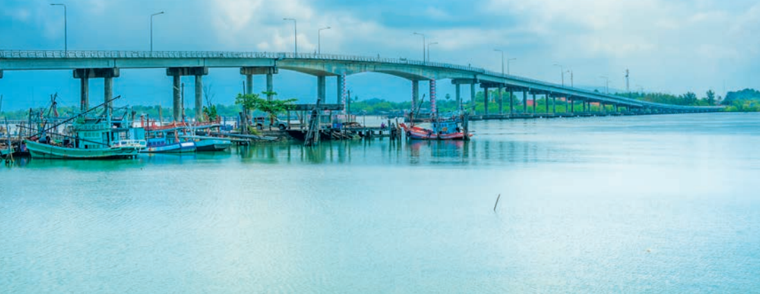
King Taksin the Great Bridge or Laem Sing Bridge
